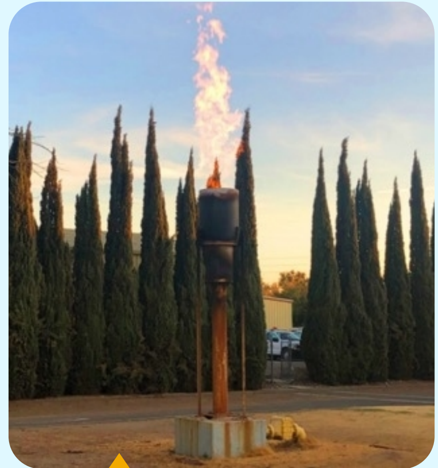
Existing Biogas Flare
